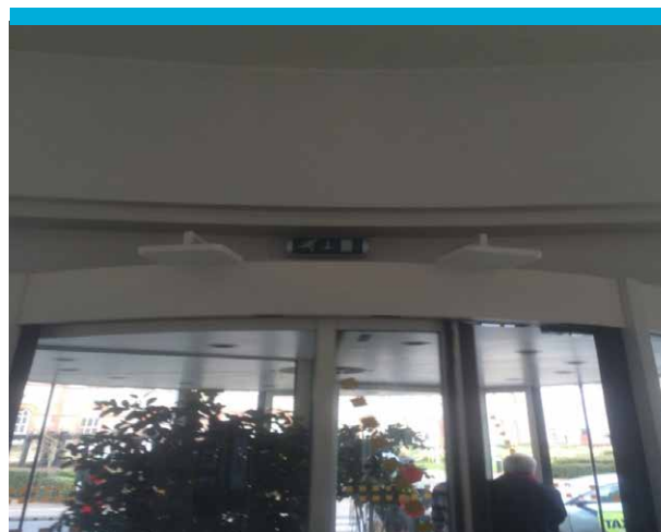
Figure 4: RFID readers installed at doors in the hospital.
