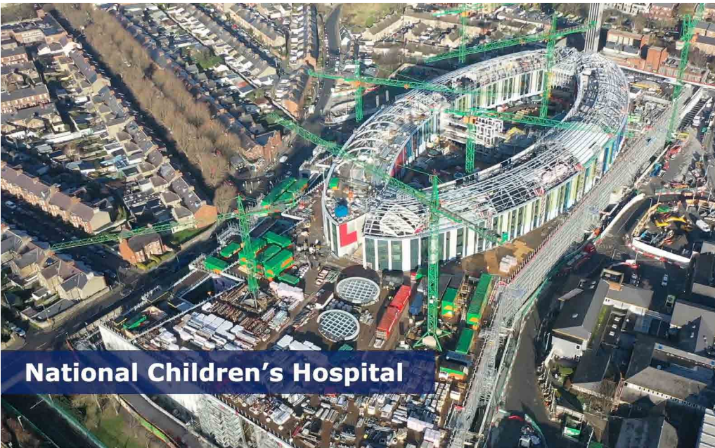
Figure 14: National Childrens Hospital, Dublin
